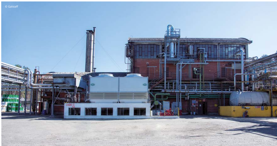
The Mornago plant.
